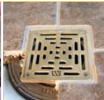
Fig 3: Cast Drain with Nickel-Bronze Strainer
