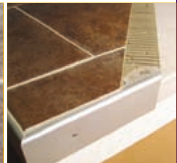
Fig 4: Pre-Finished Metal Drip Edge
